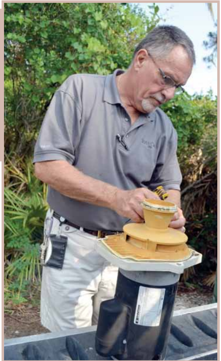
Bob Semple repairs one of the motors for the water fountains at S.R. 56 / Ancient Oaks Blvd entrance.
